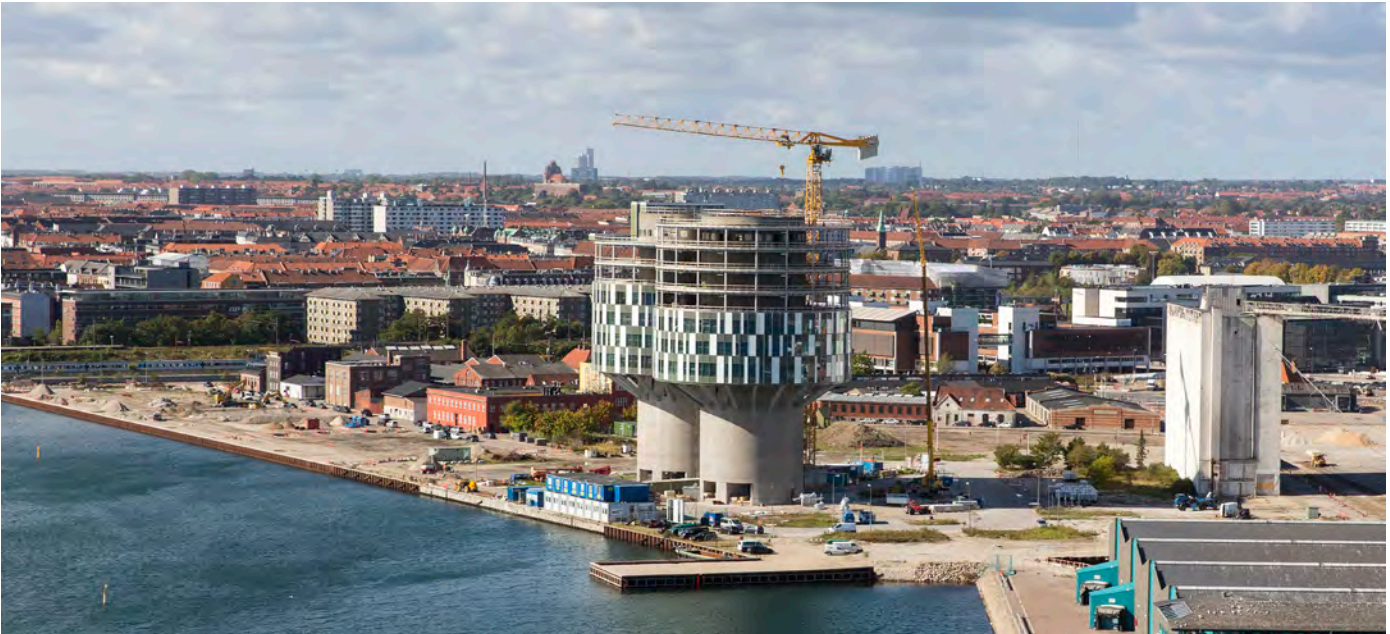
Exhibit 8: Construction of the first phase is underway. One of Nordhavnen's iconic buildings wraps residences around the concrete structure of disused smokestacks.
